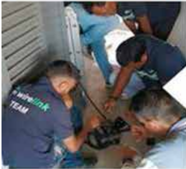
FIBRE FUSION SPLICING WORKS
