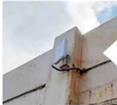
PTP WIRELESS LINK WORKS
